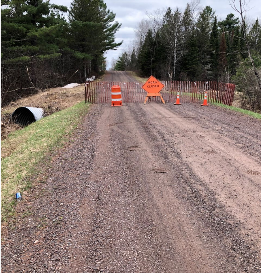
Mile and One Half Road at Mile and One Half Creek
