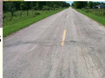
Lane Cracks/Ruts
