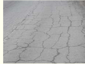
Block cracking
