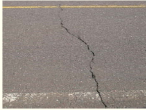
Transverse cracking
