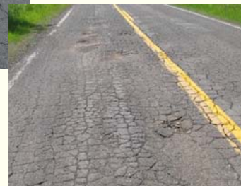
Alligator Cracking
