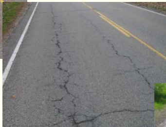
Cracking in Wheel Path
