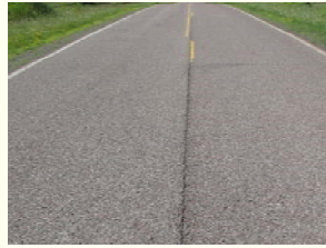
Longitudinal joint cracking
