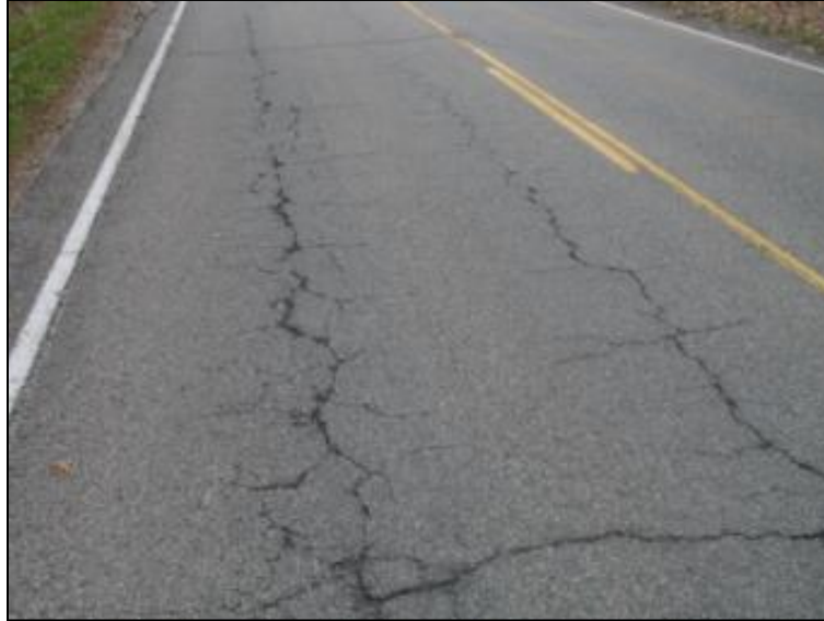
Shear Cracking
