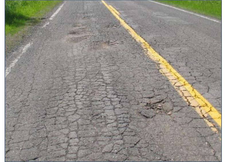
Alligator Cracking
