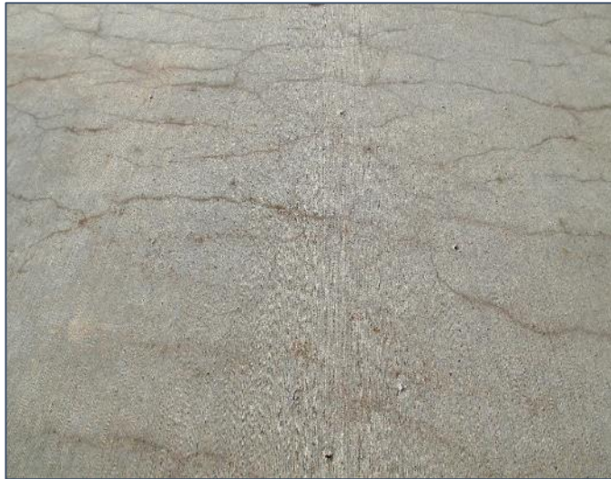
Map Cracking
