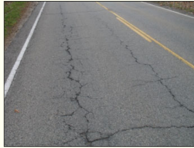
Shear Cracking
