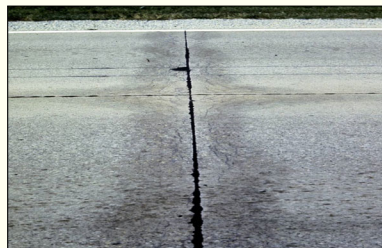
Durability Cracking
