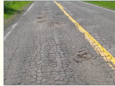
Alligator Cracking
