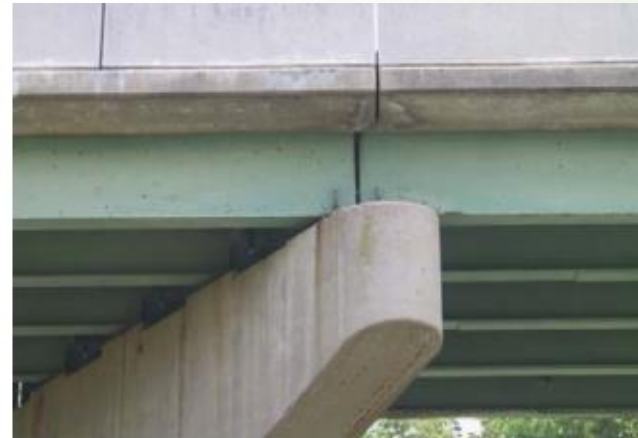
Open concrete joint used by bats
