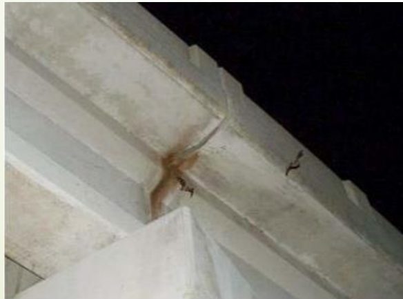
Staining on underside of expansion joint from bat use
