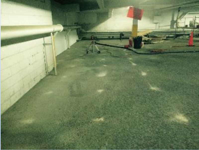
City of Ann Arbor Parking Structure Void Fill
