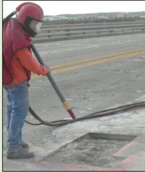
Abrasive blast cleaning of reinforcement
