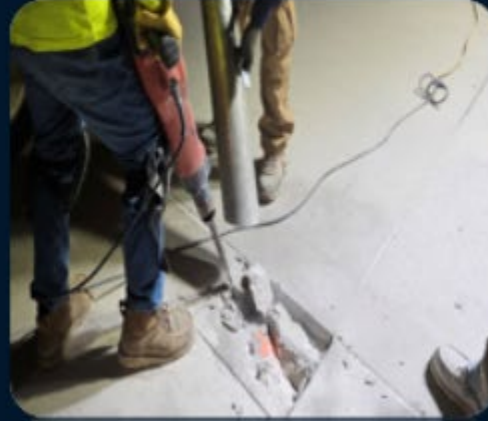
3 rd chip and vacuum to remove loose concrete
