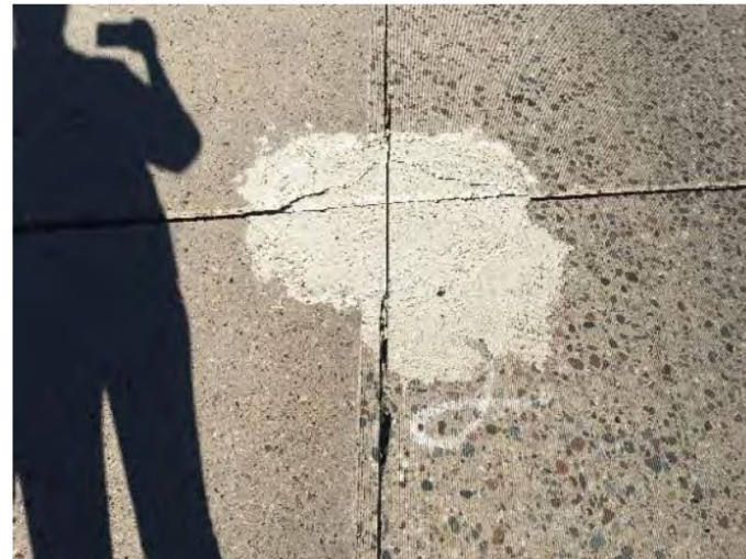
Figure 4.3 Patch Condition Rating = 3 [Linear cracks]
