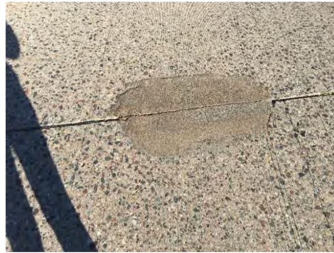
Figure 4.2 Patch Condition Rating = 4 [No Distress]
