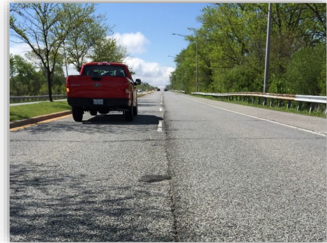
IDOT IL-50 VRAM section at 14 yr old
