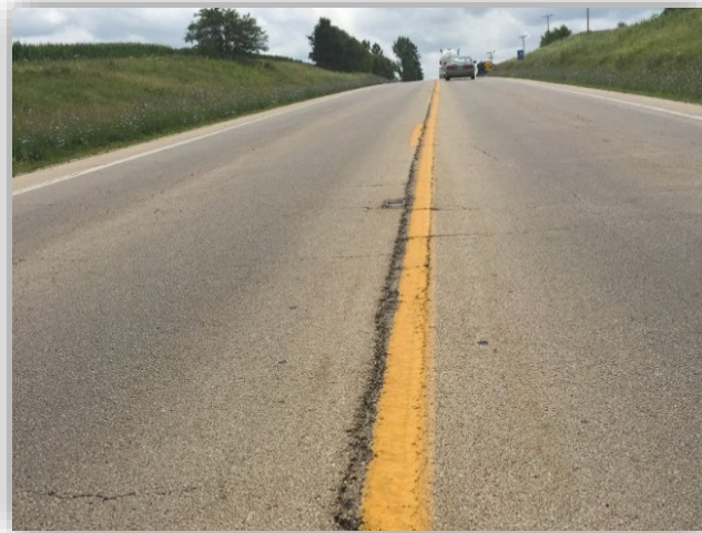
IDOT IL-26 VRAM section at 14 yr old
