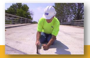
1. Identify and remove unsound concrete and existing thin polymer concrete overlay (thick, structurally sound overlays may remain)
