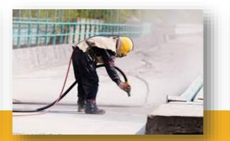
2. Abrasive blast all substrate surfaces. Clean by shotblasting.
