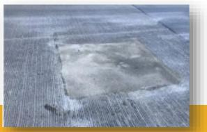
3. Use PPC 1121 or HCSC to patch substrate concrete for optimal compatibility with the existing deck as the TPO AD base.
