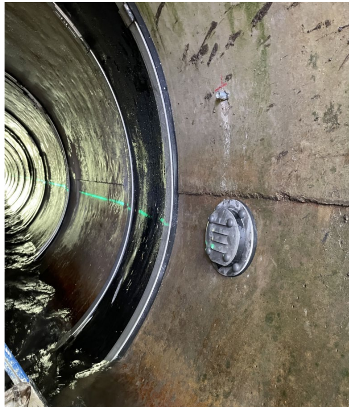
Jet Filter Install
