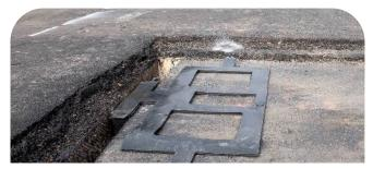
In-road charging system made of under-road coil segments.
