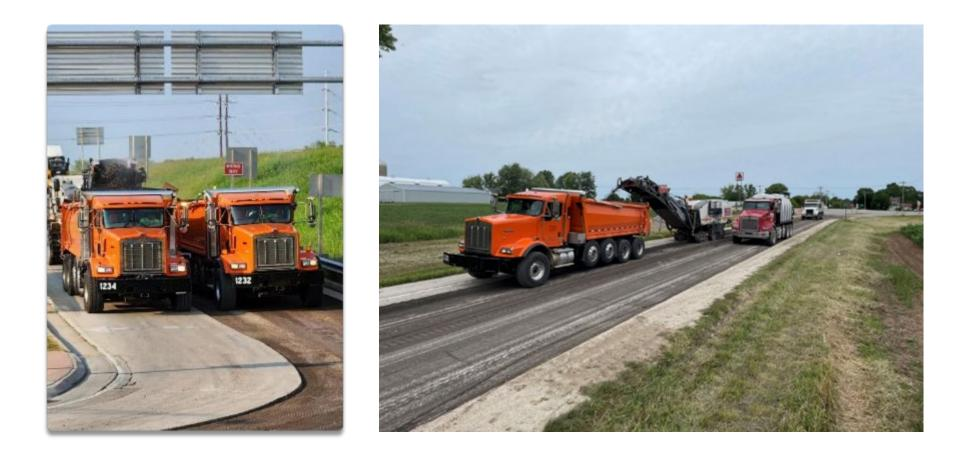
Milling projects utilizing the construction method to increase center crown to a Sheboygan County standard of 3 percent allow proper drainage.
