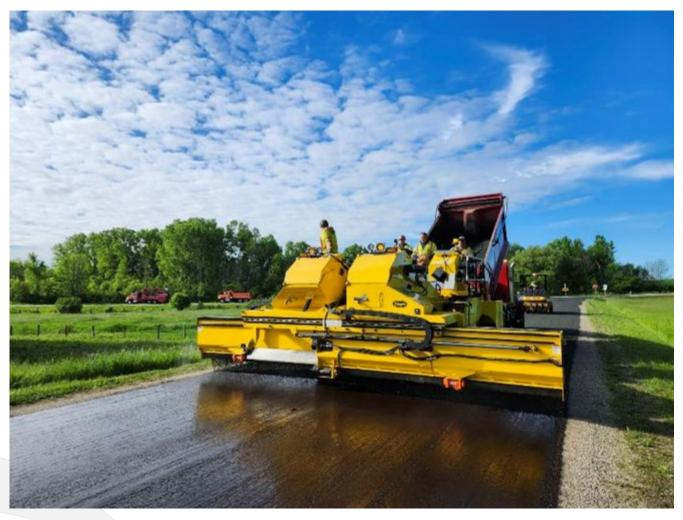
In 2024 – 30 miles of county trunk highway was chip sealed using a 100 percent fractured <u>black granite stone</u>.
