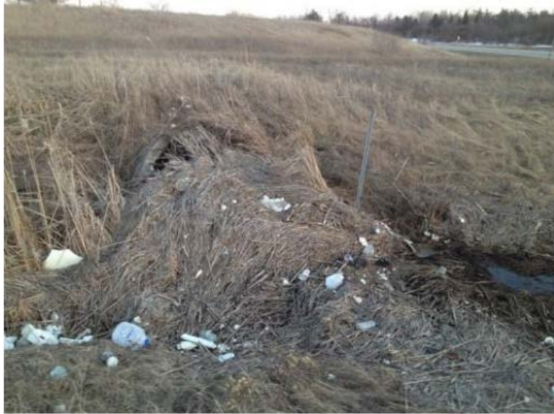
Figure 8.2.17: Blocked inlet
