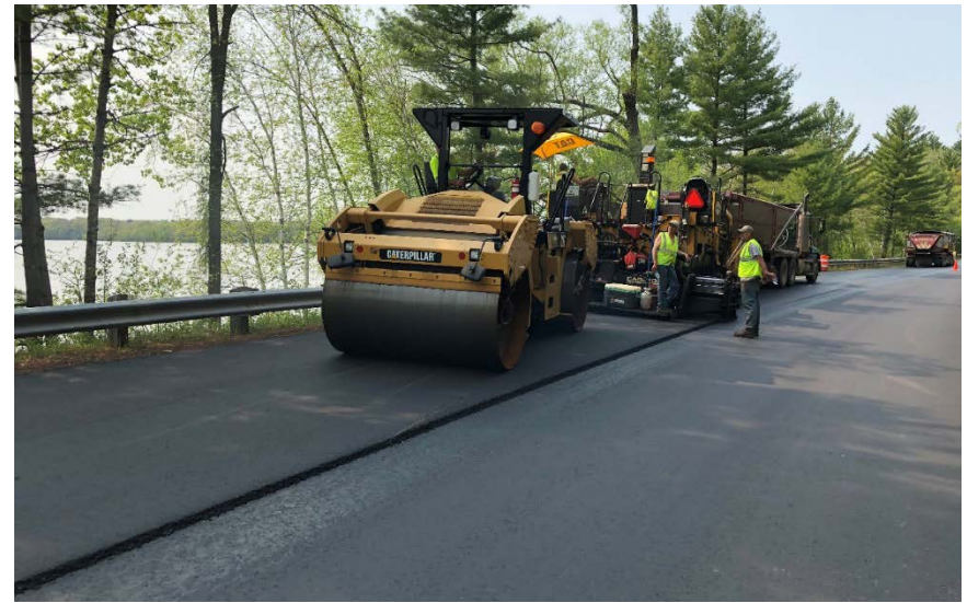
Surface layer placement
