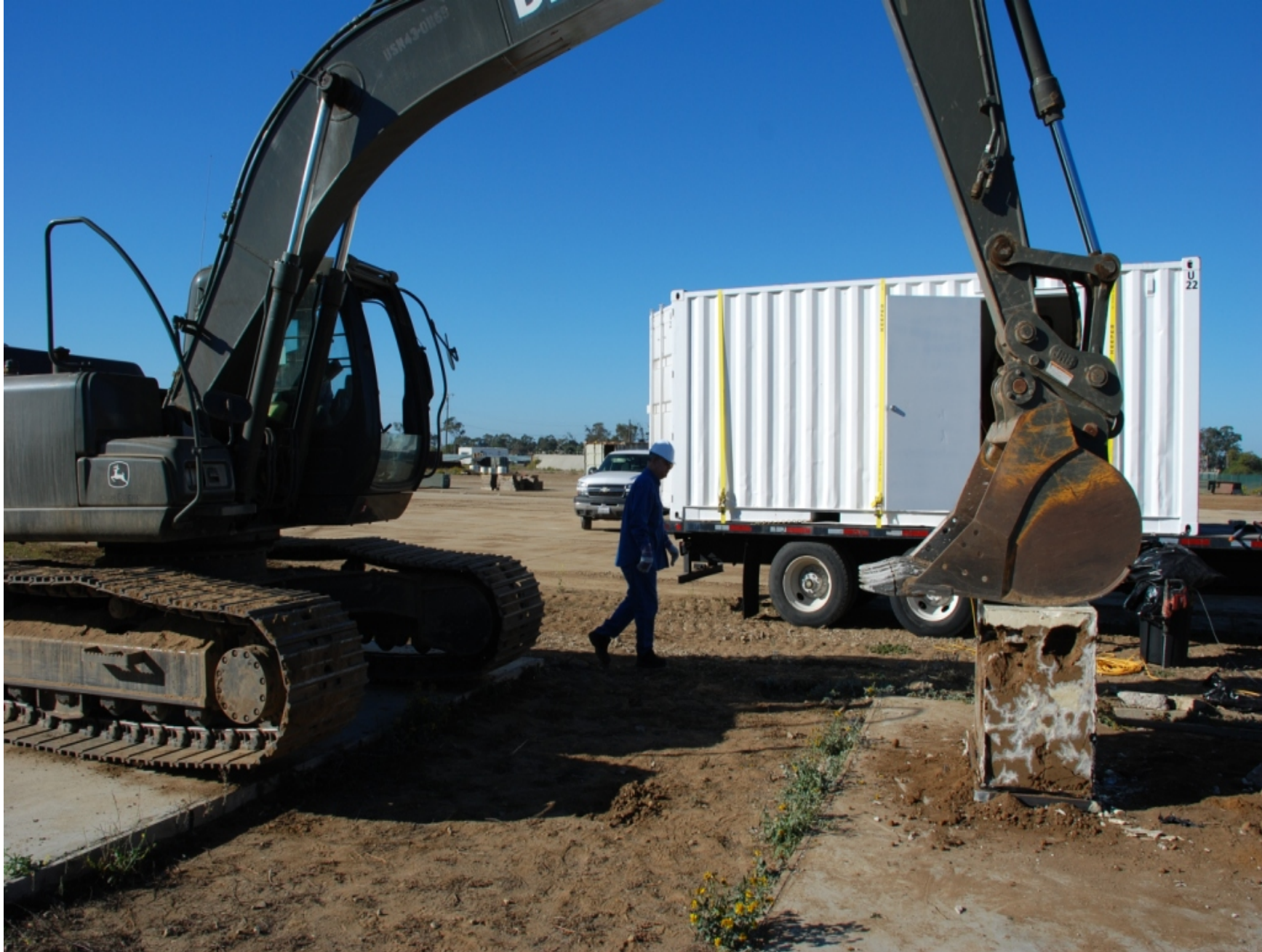
Vertical load applied using an excavator
