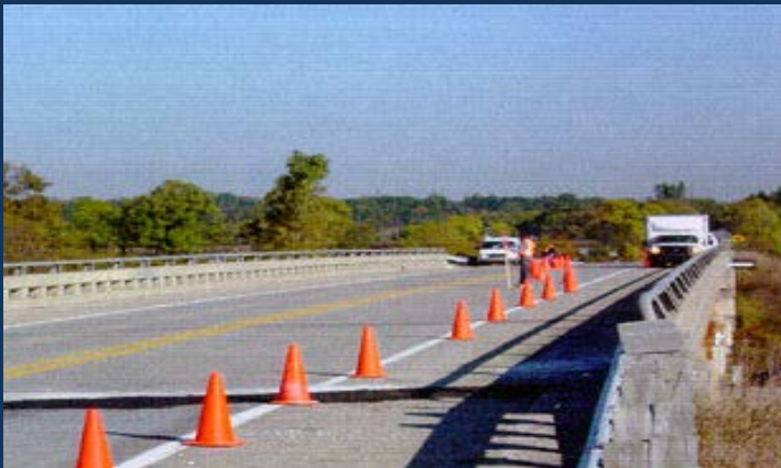
Curtis Road Bridge, Michigan
