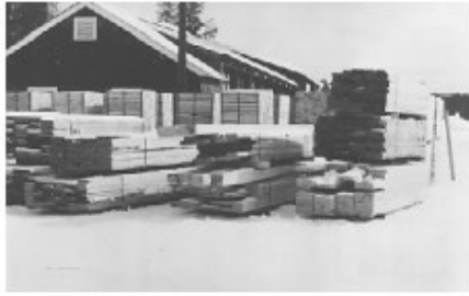
Figure 5—Eastern Hemlock lumber for the Big Erick's bridge awaiting preservative treatment.
