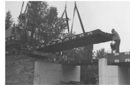
Figure 9—Placement of half-width panels with an overhead crane.
