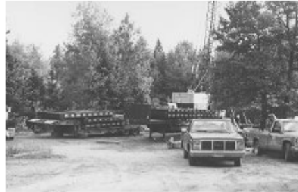
Figure 8—Prefabricated half-width panels arriving at the bridge site prior to installation.
