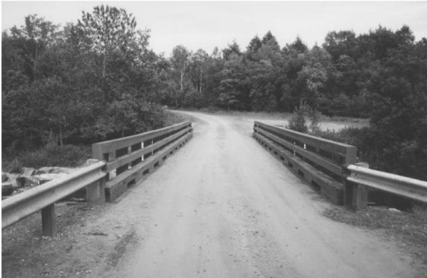
Figure 12—Completed Big Erick's bridge: side view (top), end view (bottom).
