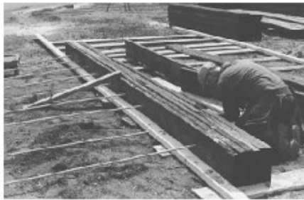
Figure 5—Eastern Hemlock lumber for the Big Erick's bridge awaiting preservative treatment.
