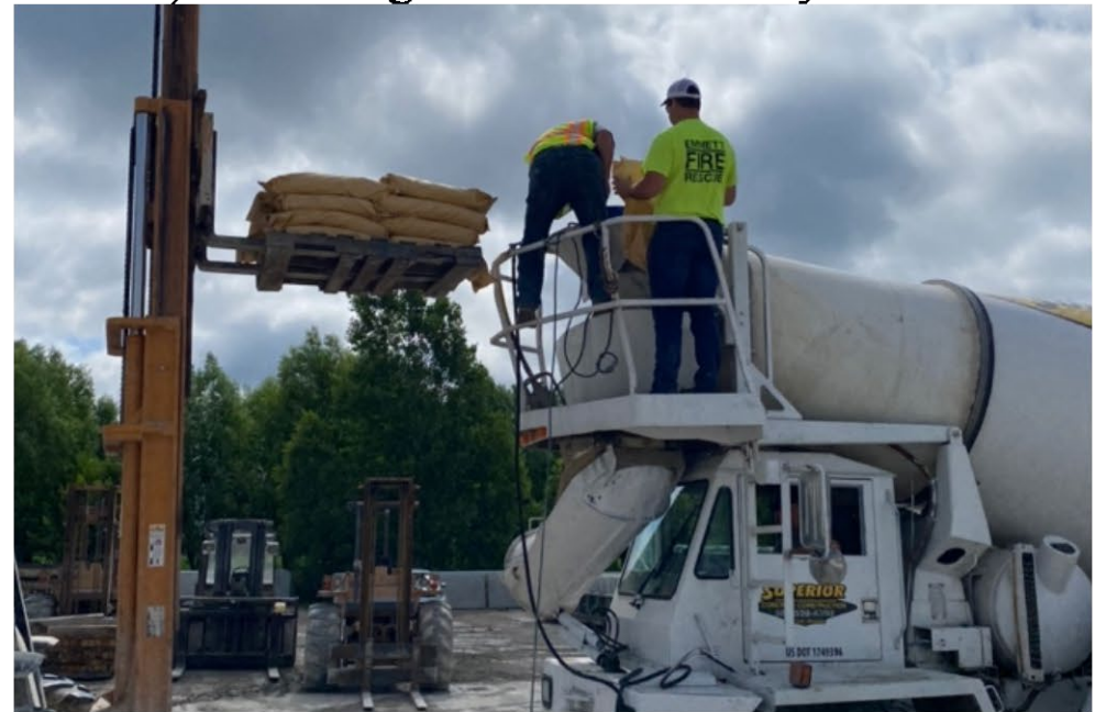
d) Loading steel fibers
