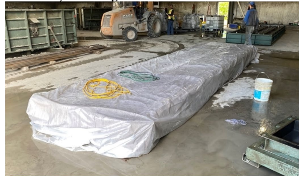
d) Wrapped and curing panel
