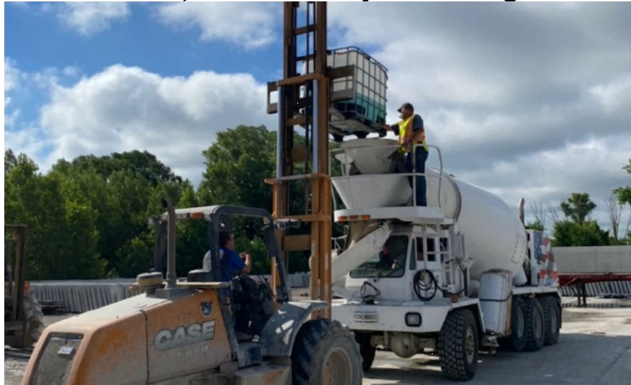
c) Loading of water and water reducer
