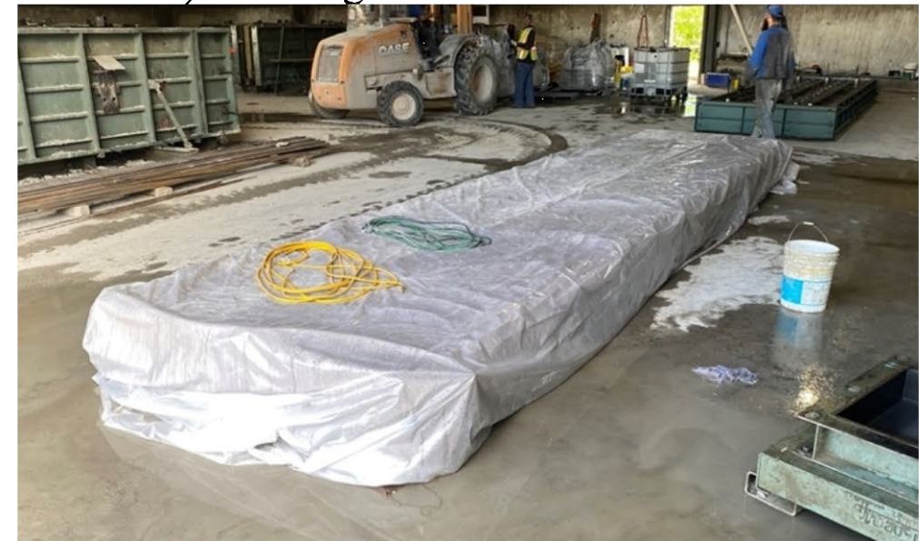
d) Wrapped and curing panel
