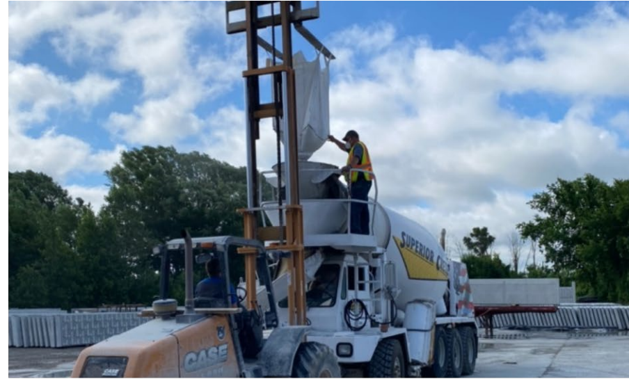
b) Loading of sand into ready-mix truck
