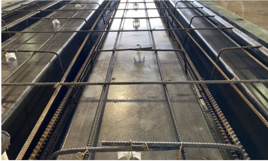
a) Forms ready for casting
