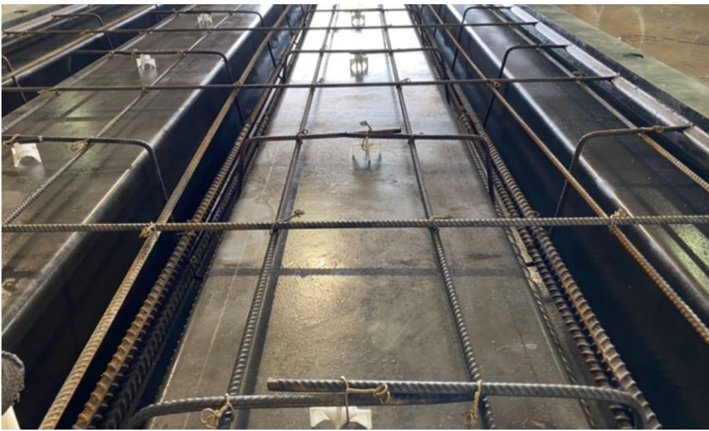
a) Forms ready for casting
