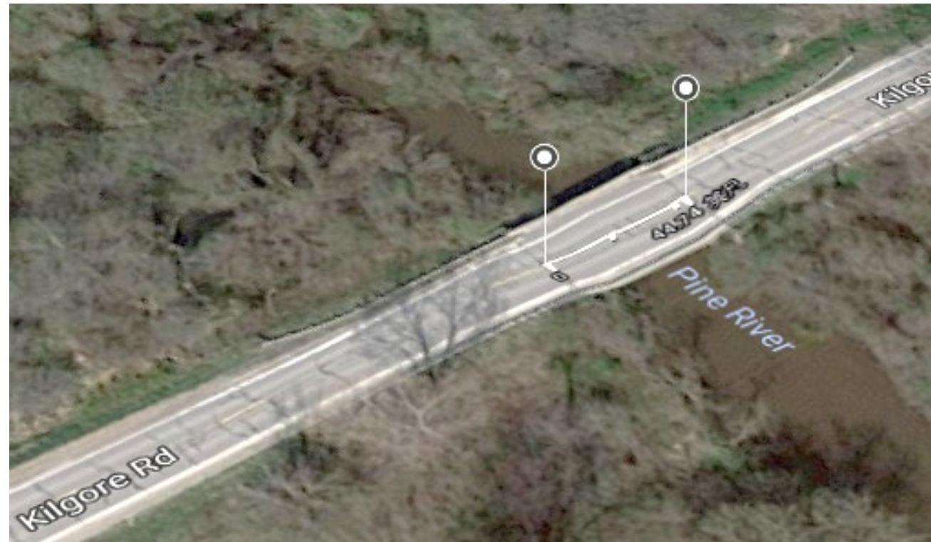
(b) Bridge site
