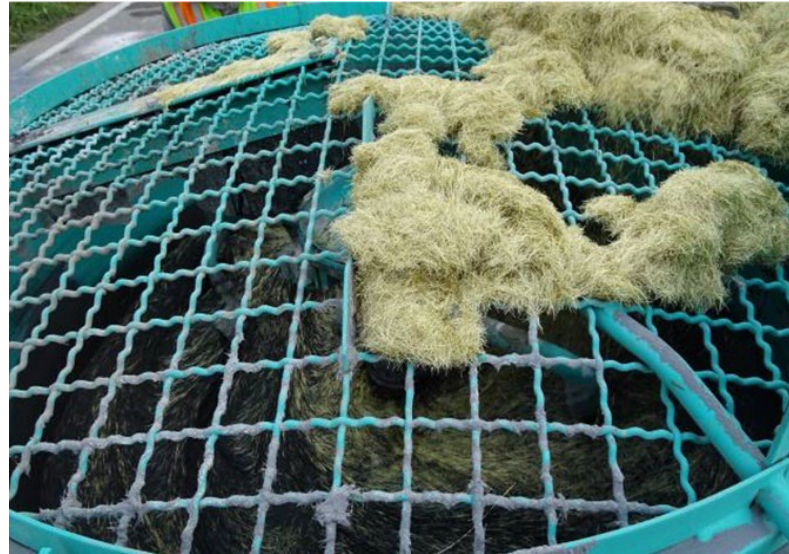
(e) Addition of steel fibers
