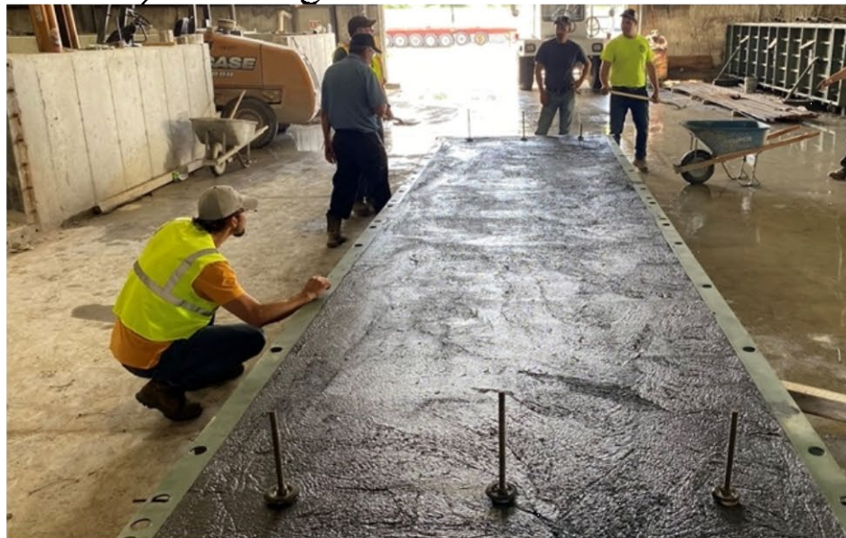
c) Finished panel
