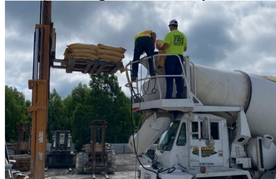
d) Loading steel fibers
