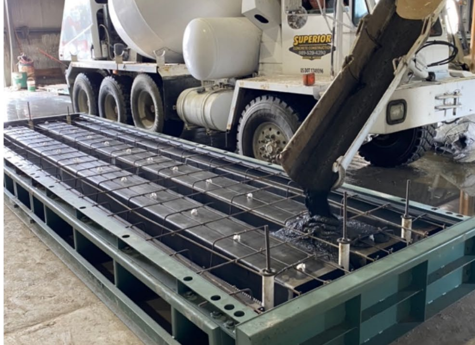
a) Casting of UHPC materials in form
