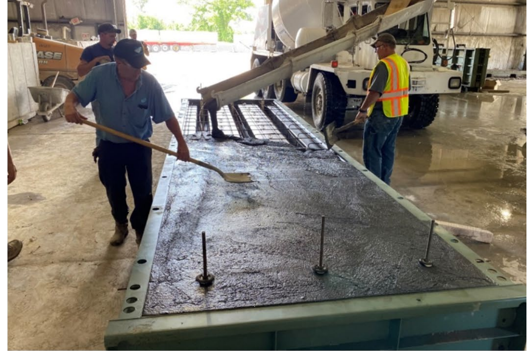
b) Casting of UHPC materials in form
