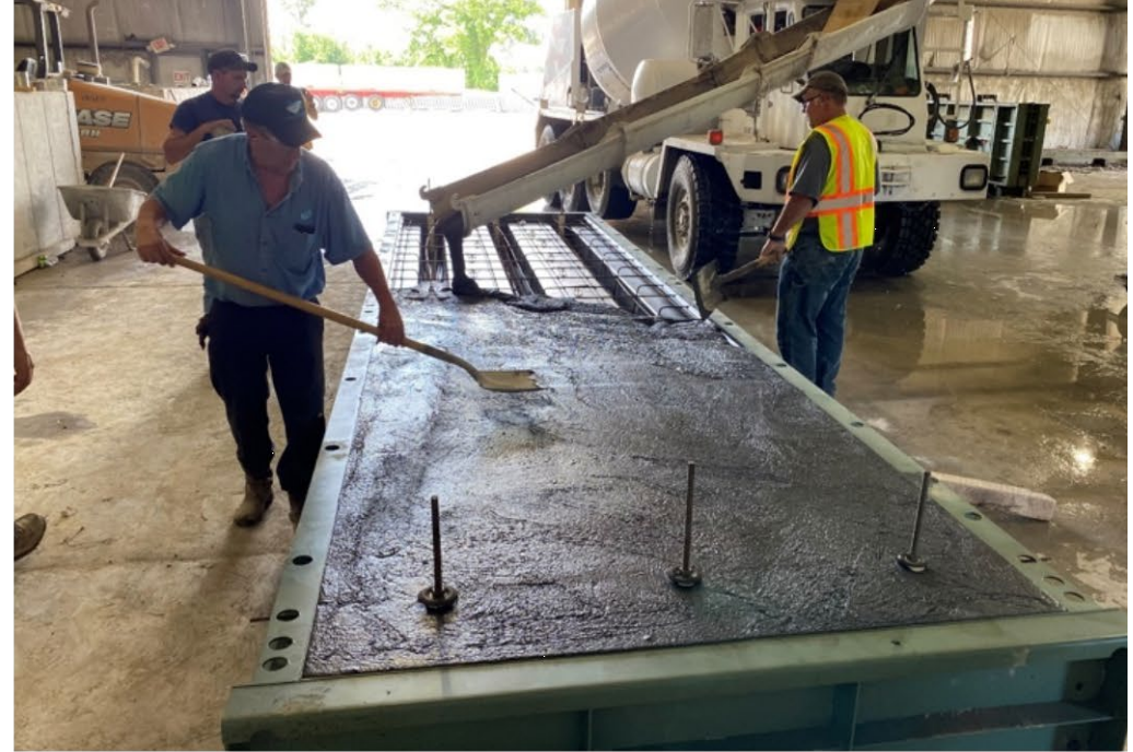
b) Casting of UHPC materials in form
