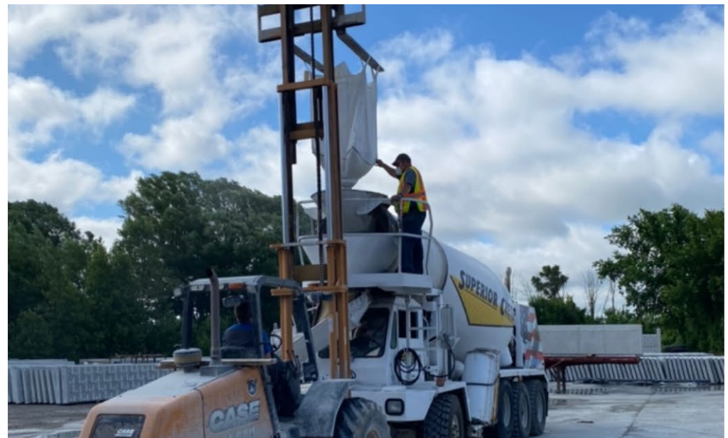
b) Loading of sand into ready-mix truck
