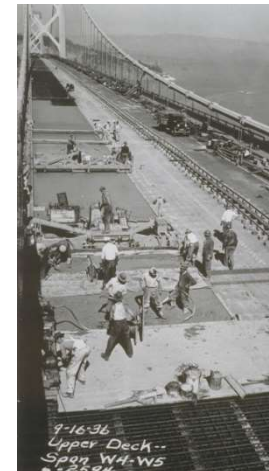
PLATE No. 4.—The bridge will have two decks. The top deck will have six lanes for passenger automobiles; the lower deck will have three lanes for trucks and buses—it will also have two standard gauge electric railway tracks.
