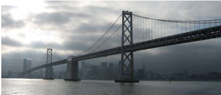
PLATE No. 4.—The bridge will have two decks. The top deck will have six lanes for passenger automobiles; the lower deck will have three lanes for trucks and buses—it will also have two standard gauge electric railway tracks.
