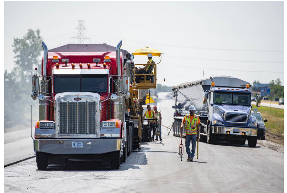
Paving on I-75 in Bay Region
