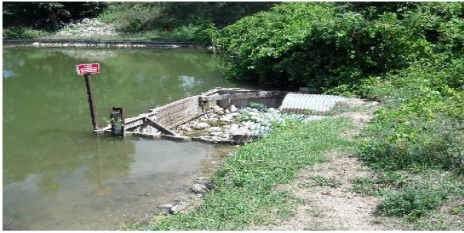
Control structure at upstream end of culvert
