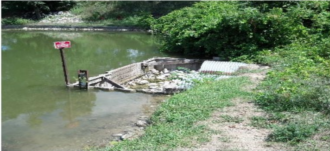
Control structure at upstream end of culverts
