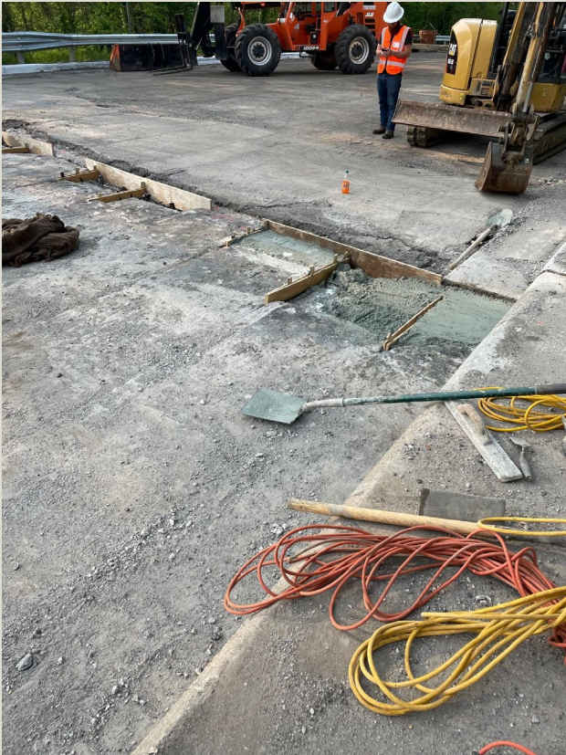
Concrete Deck Patching
