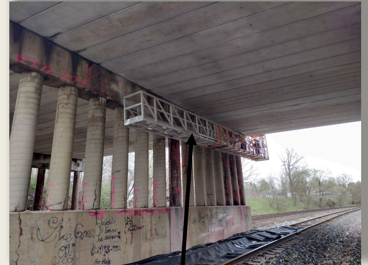
work platform underneath bridge
