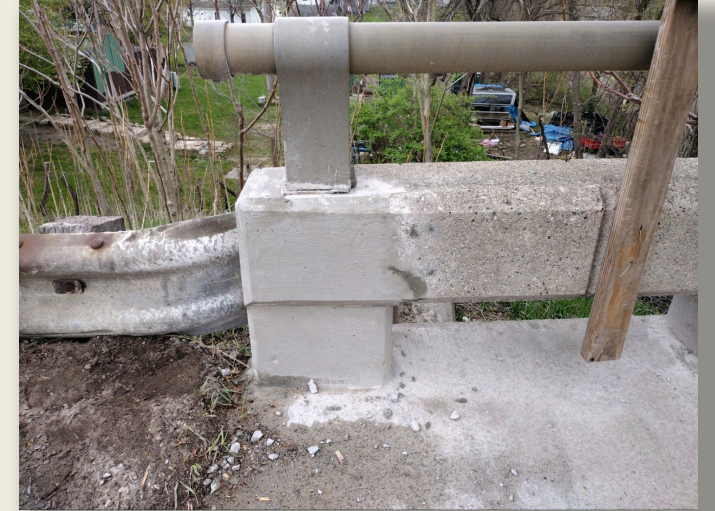
Minor Concrete Repairs
