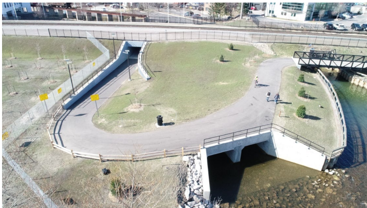
Allen Creek Berm Opening
