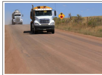
Stable fines preservation on a treated road
