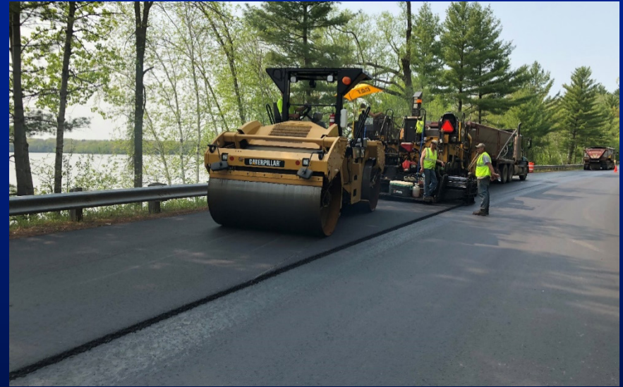
Surface layer placement
