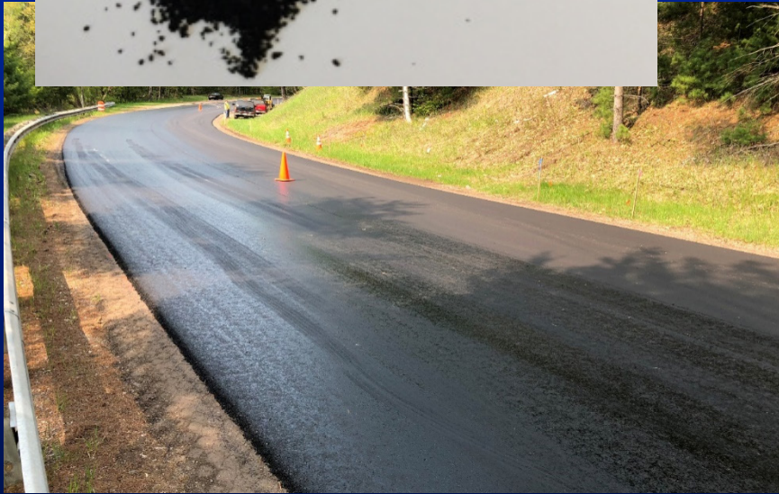
Emulsion application before surface placement
