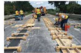
Figure 7. Photo. Installation of UHPC connection repair project on the Kilgore Road Bridge over Pine River in Keweenaw Township, MI.
