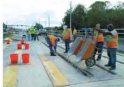
Figure 6. Photo. Installation of UHPC on one of the Martin Downs Boulevard Bridges.
