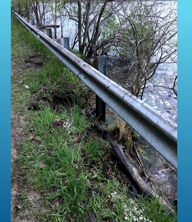
OCRC INSTALLED GEO TECH FABRIC AND 21AA LIMESTONE AS TEMPORARY MEASURE
