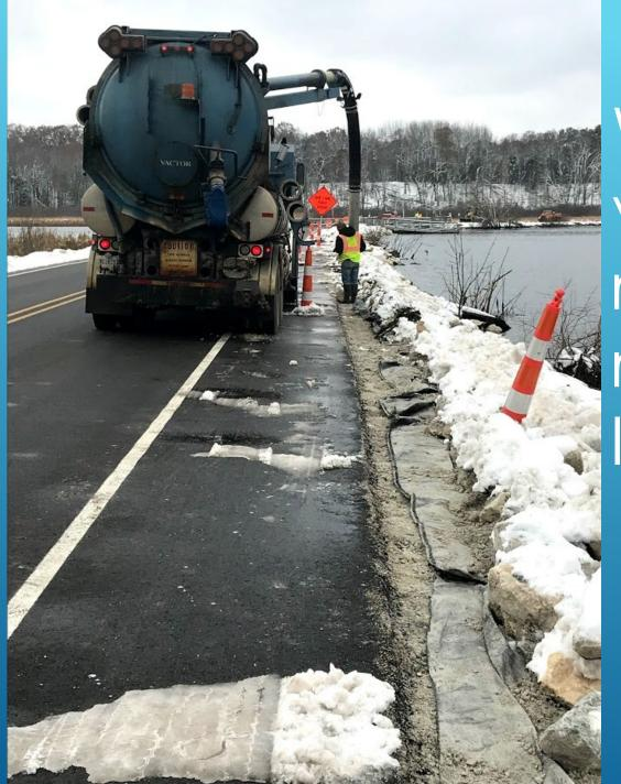
We then used vac truck to remove remaining limestone
