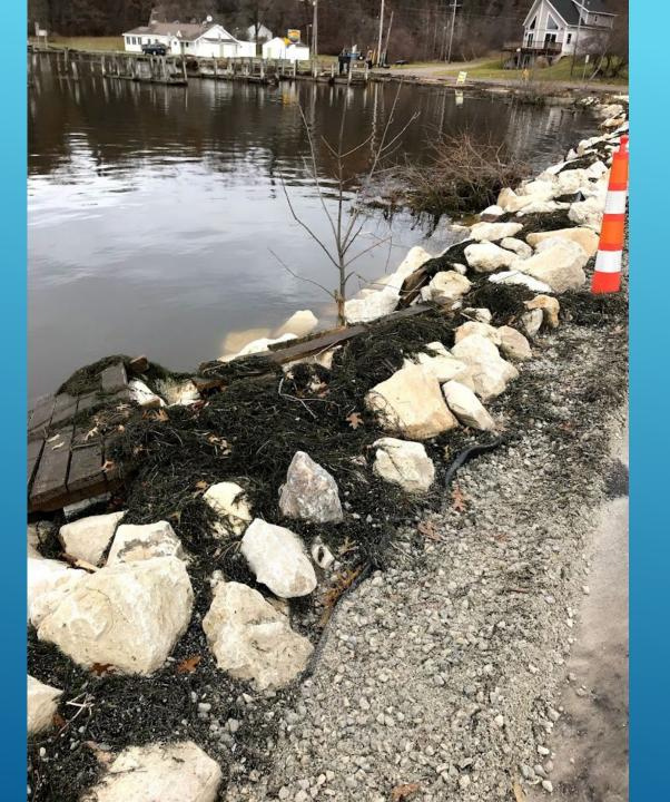
**ORIGNIALLY** WE PLACED 21AA LIMESTONE ON **SHOULDERS BUT WAVE** ACTION **WASHED IT** OUT
