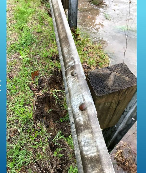
STORM FROM EAST CAUSED **EROSION** THAT THREATENED TO WASH OUT ROAD
