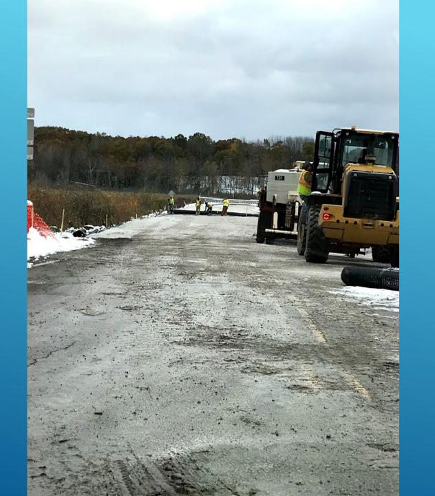
BRINE TRUCK TO KEEP AGGREGATE FROM FREEZING
