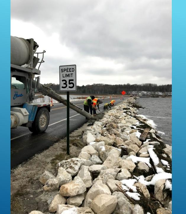
WE THEN **POURED** CONCRETE BETWEEN **ASPHALT** SHOULDER AND RIP RAP
