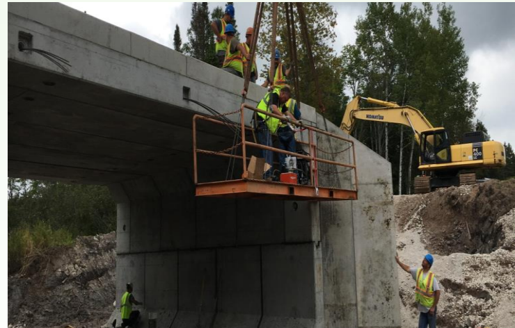
Post-Tensioning all units together
