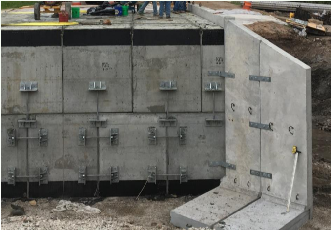
Pre-Cast Headwall and Wingwalls
