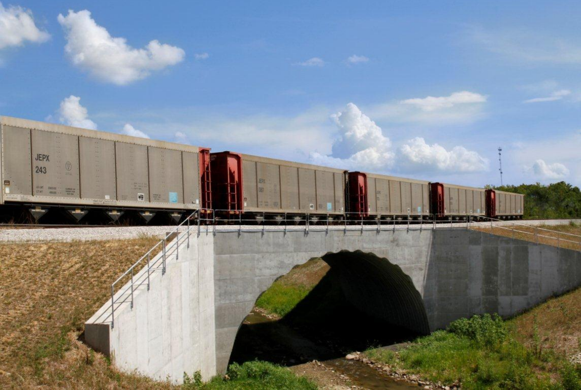
Knox County, Indiana E-80 Cooper Engine, 52.5 ft span
