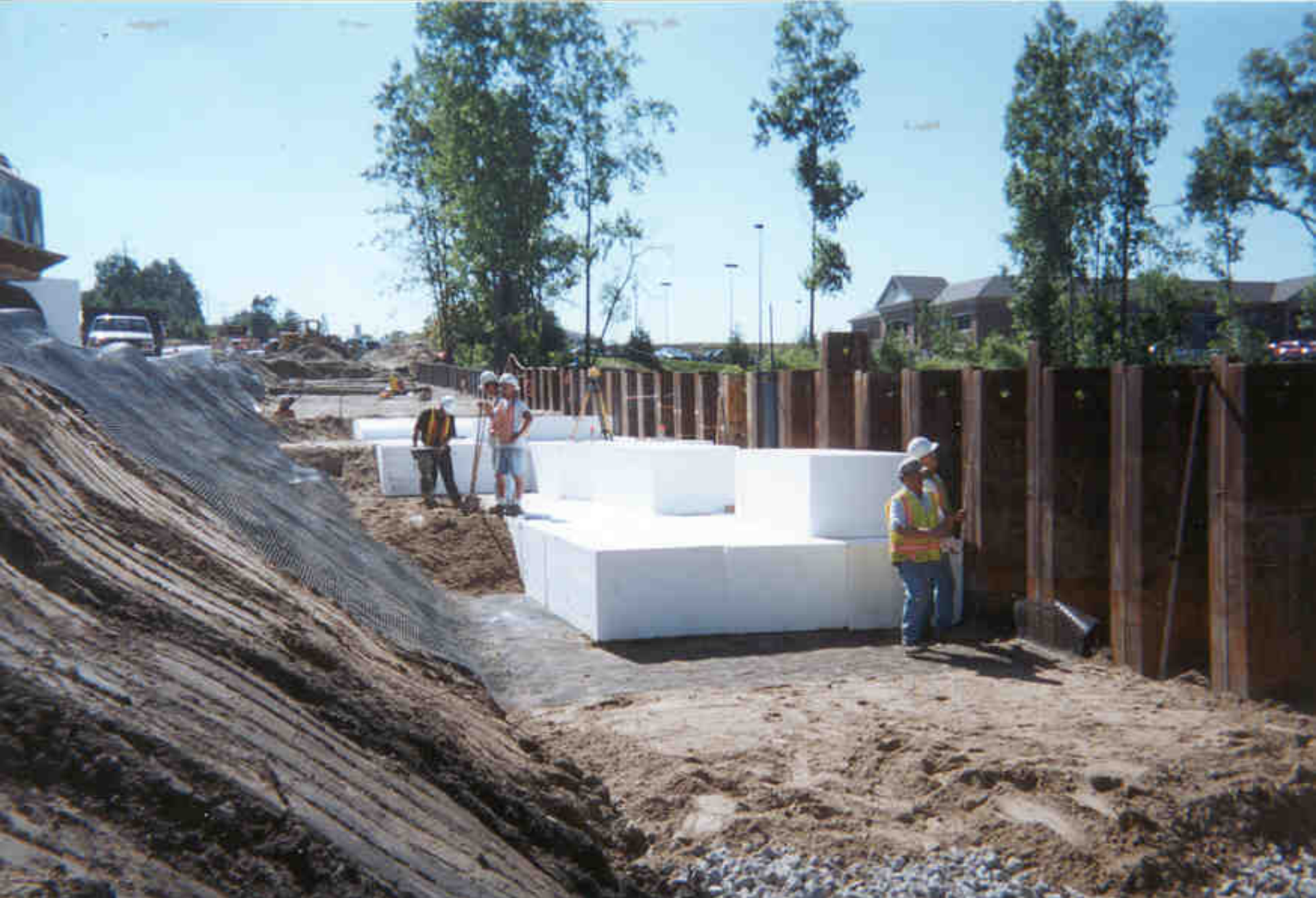
Placement of EPS and Geogrid behind sheeting.
