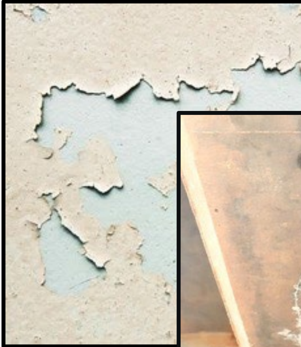
Flaking paint/stucco on walls
