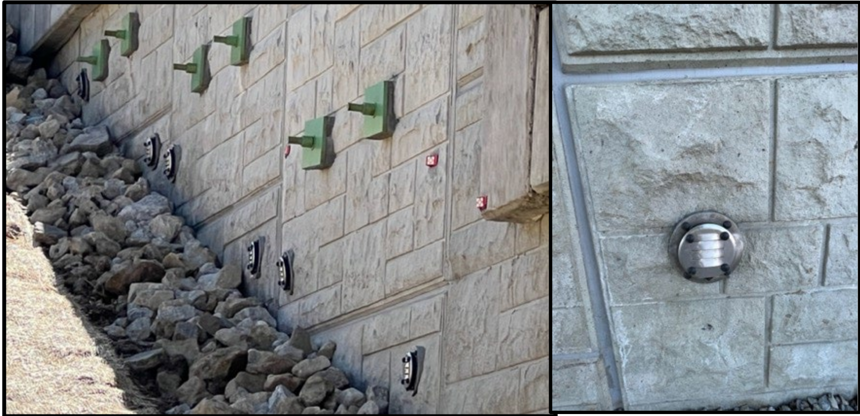
Kenilworth Road over US 31 St. Joseph Co.
