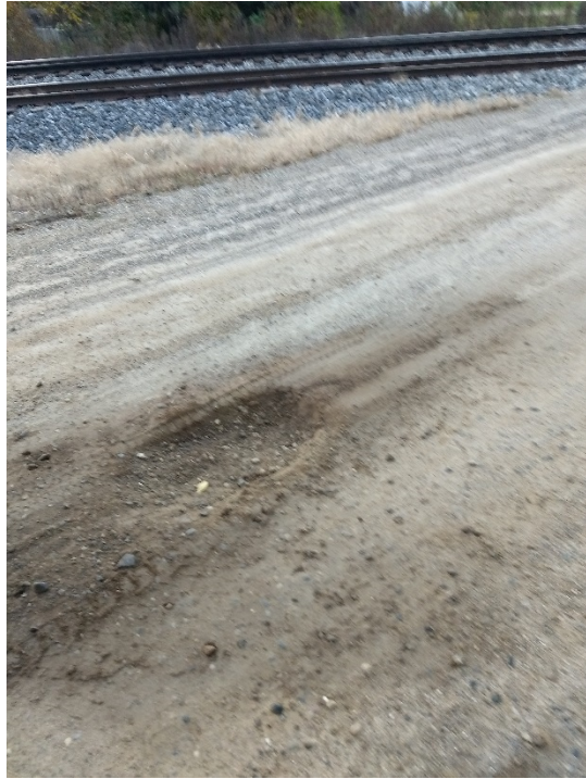
Poor Subgrade
