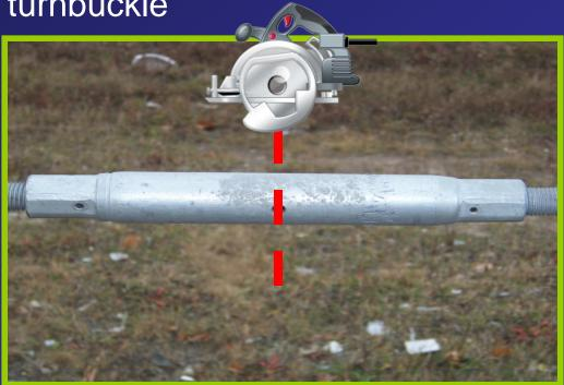
Before cutting turnbuckle, it is desirable to remove adjacent posts in the vicinity of the turnbuckle
