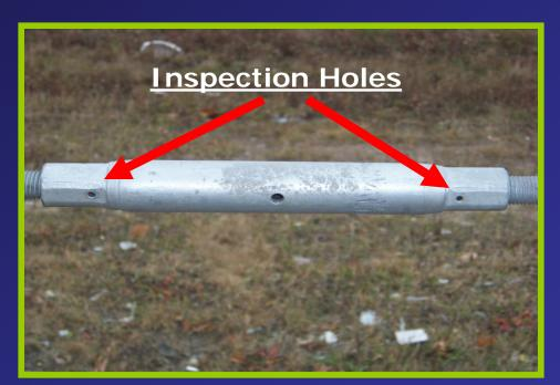
**Note:** Check both inspection holes while loosening turnbuckle
