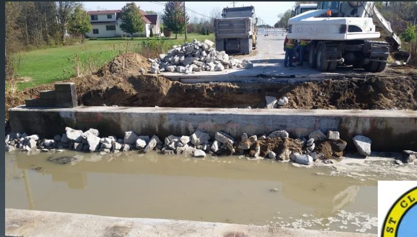
Riprap for Scour Protection
