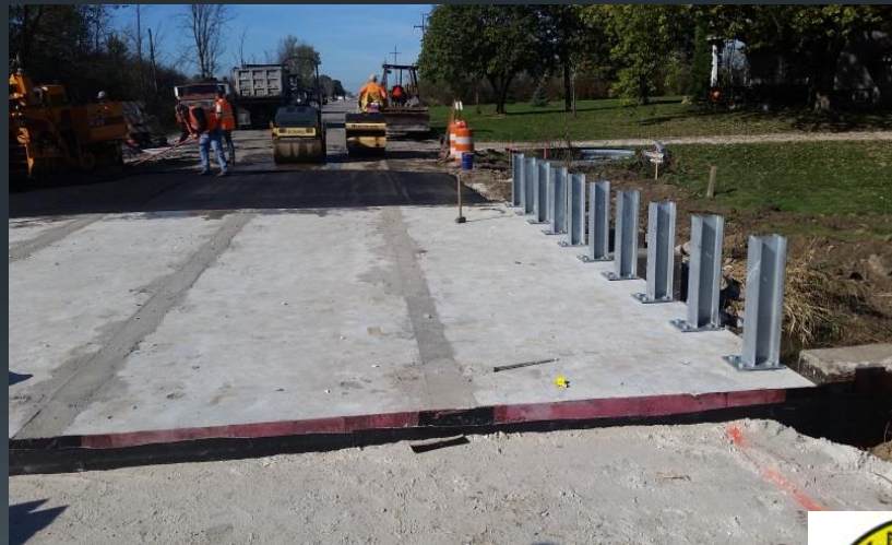
Install Guardrail Posts
