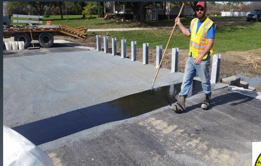
Cover with Aggregate and Re-Epoxy
