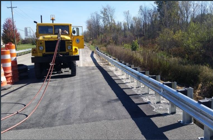
Install Guardrail
