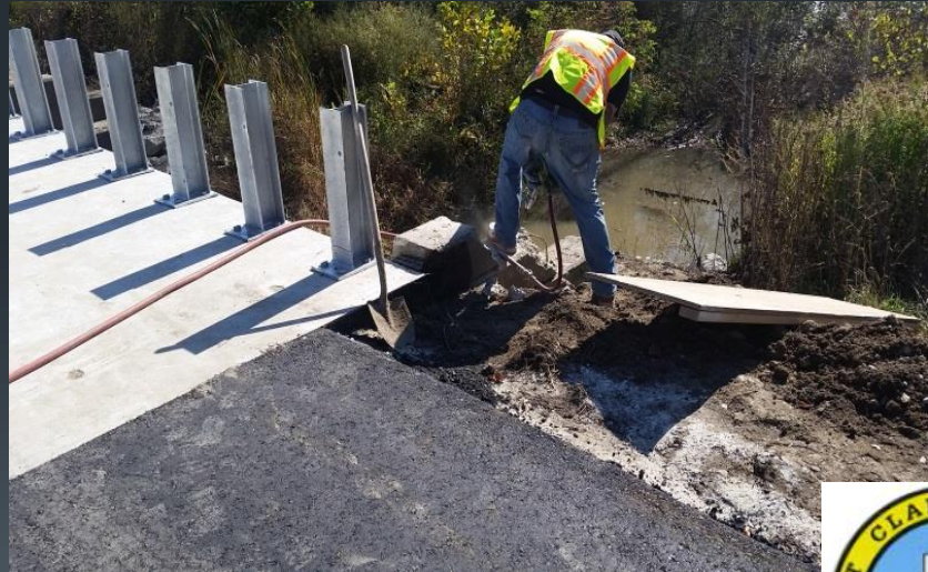
Repair Existing Wingwalls
