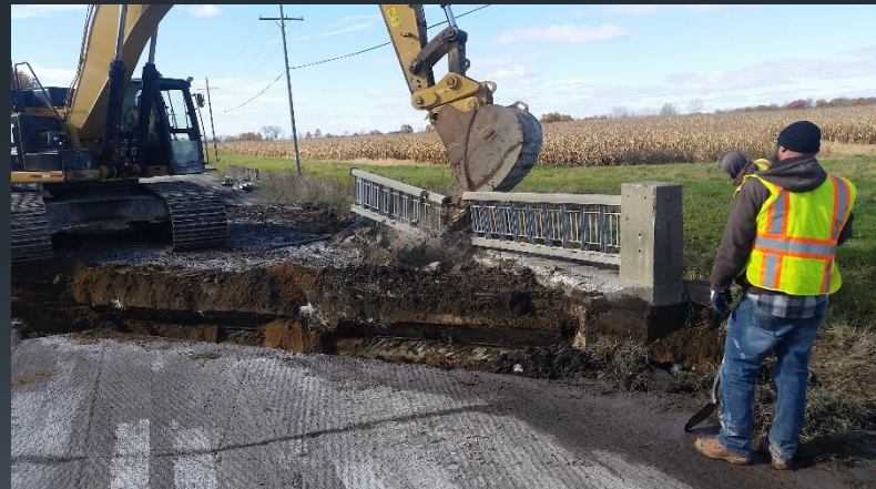
Existing Substructure to Remain
