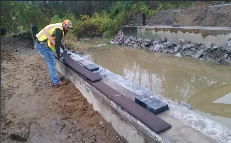
Bearing and Joint Filler
