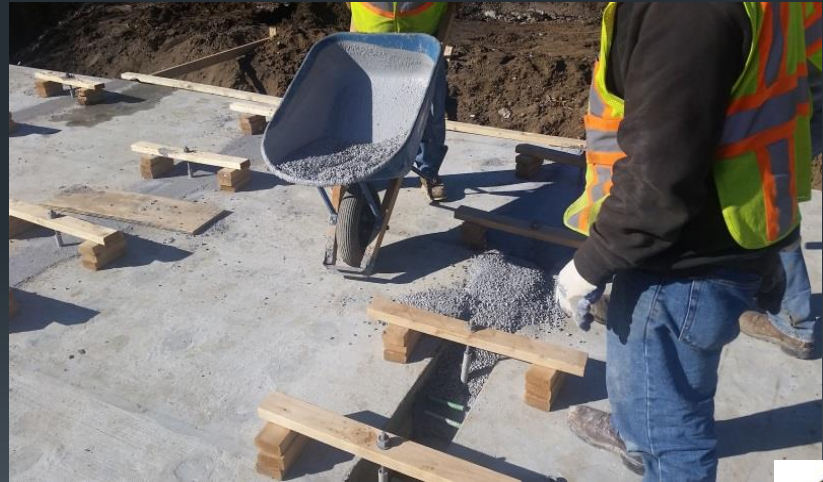
Pouring T-17 Polymer Joint Concrete
