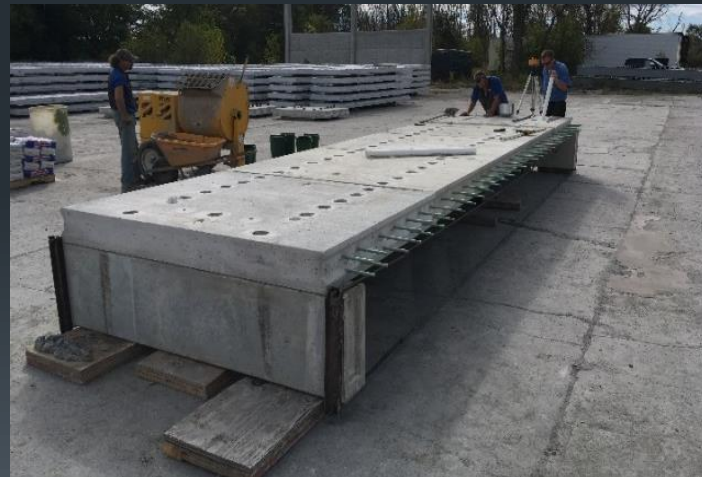
Fabrication of Bridge Unit
