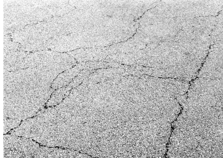
Block Cracking
