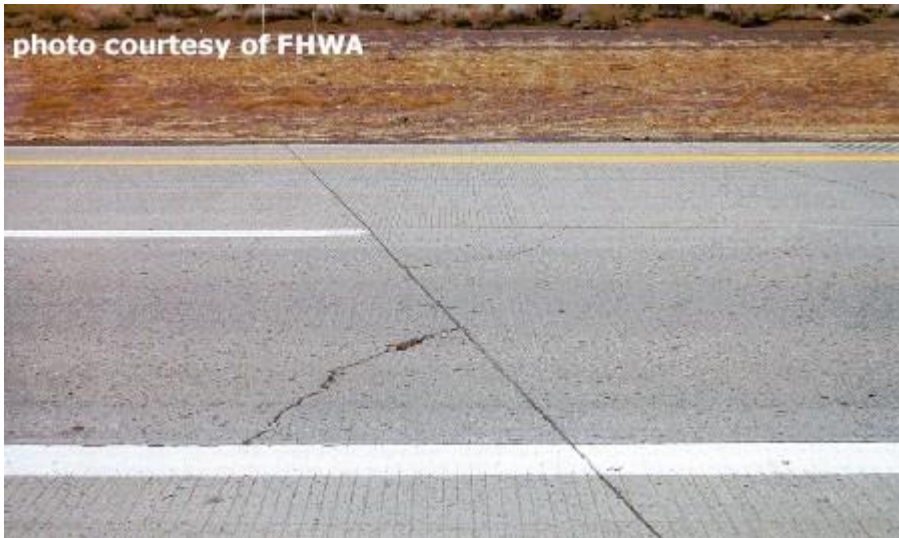
Corner Cracking
