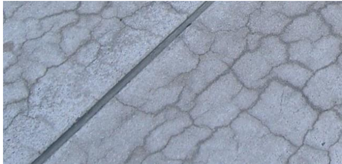
Map Cracking
