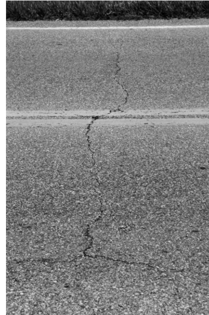
Transverse Cracking
