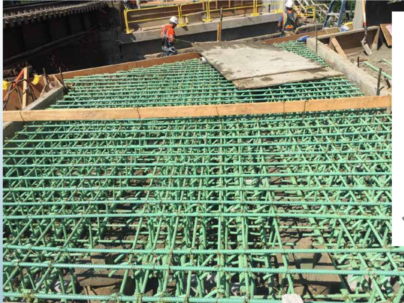
Approach Slab Installation
