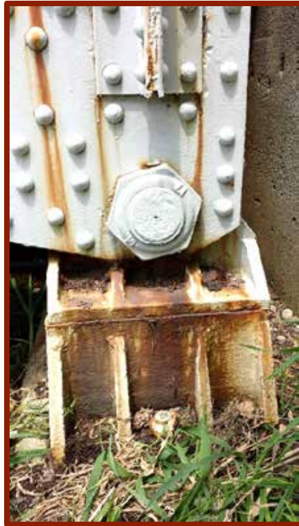
Fixed bearings before and after.
