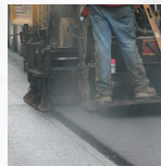
Mill and Overlay
