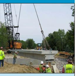
Steel tub girders offer an alternative to standard I-girders for the construction and design of bridges. Bill Hazelton, Dewayne Rogers, and Guy Nelson will be presenting on St. Clair County's experiences with steel tub girders.
