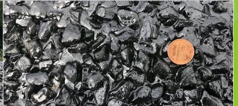
Final product with Fog Seal Application
