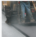
Mill and Overlay
